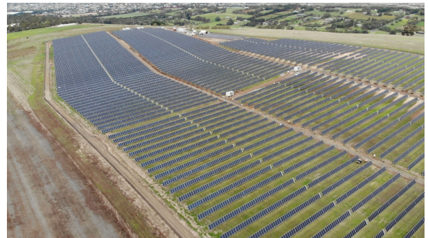
Figure 2. A distant view of the layout of solar panels on the farm
