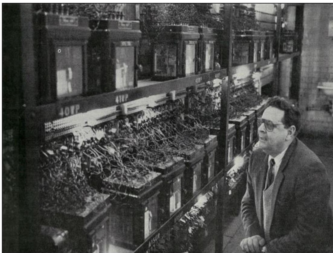
Engineering Ethics in Practice: safety-critical railway signalling equipment and wiring in a dubious state of serviceability. Did anyone blow the whistle? (Photo: courtesy The Age )
