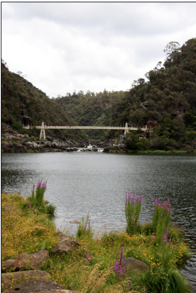
WILDFLOWERS, white-water, and wide span pedestrian bridge, Central Tasmania.
