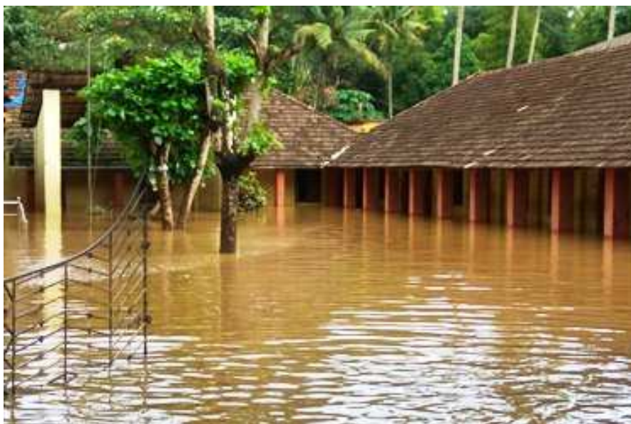
Figure 1: School immersed in water damaging computer lab and other electronic equipment.
