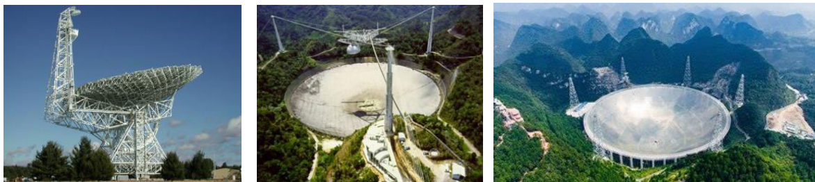
Figure 7 : the picture on the left is of the largest fully steerable single dish radio telescope in existence today – the 100-m Greenbank Telescope in USA; the other two are largest non-steerable (fixed) single dish radio telescopes : the 300-m Arecibo Radio Telescope (middle) in Puerto Rico, and the 500-m FAST observatory (right) in China
